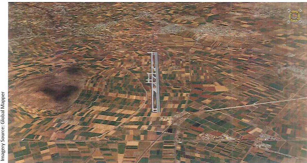
Figure 19. Tepeji del Río Northeast-Southwest Runway (View from the Southwest)
